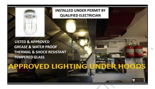
Lighting used for hoods must be listed, approved and installed in accordance with the listing and manufacturer's instructions. Lighting units should be equipped with tight fitting protective globe lights with steel enclosures that are mounted on the outer surface of the hood. All electrical equipment should be installed in accordance with the electrical code by a licensed electrician with a permit from the electrical authority.
