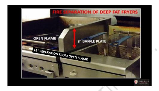
All deep fat fryers must be separated from flames from adjacent cooking equipment by at least 16". If a steel or tempered glass baffle with a minimum height of 8" is installed between the fryer and the adjacent appliance the requirement for the 16" separation is waved.
