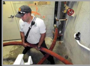
5 YEAR WATER FLOW AND PRESSURE VALVE TEST
