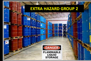
FLAMMABLE & COMBUSTIBLE LIQUID STORAGE
