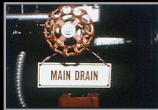
MAIN DRAIN TEST
