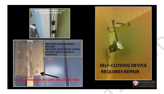
When assessing the operation of a door carefully examine all parts including the door leaf, frame, hinges, latching device, handles and the threshold. Over time things like loose or missing screws in the hinges can impede the proper operation of the door.
