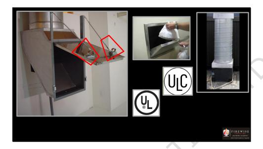
The bottom of the chute is equipped with a discharge door protected by a fusible link that will melt in case of a fire in the discharge room. Once the link melts the door must automatically close to seal off the chute. This is a simple mechanism but vital to the safety of the building. Normally, the discharge door is kept in the open position so trash will not accumulate in the shaft causing a fire hazard.
