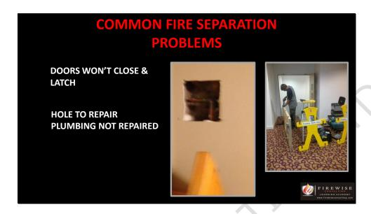
There are a number of common problems with fire separations. Doors won't close and latch or they are wedged in the open position. Holes in walls and ceilings that are part of the fire separation are made to repair plumbing or electrical problems but the holes are not repaired. Holes that are not repaired allow fire to travel into concealed spaces making it very difficult for firefighters to locate and extinguish the fire.
