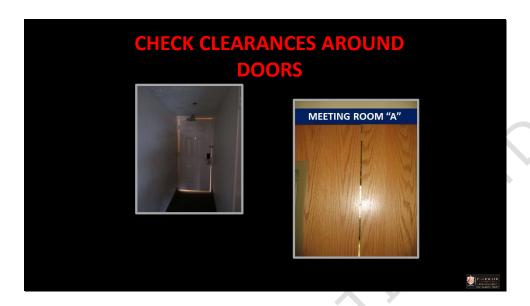
Check the clearances around the door top, bottom and sides to ensure there are no large gaps that would allow the spread of smoke and hot gasses in the event of a fire. If you can see light between the door and the door frame clearance issues are likely and the door may need adjustment. The same is true for double door configurations. Only a minimal clearance should be present.
