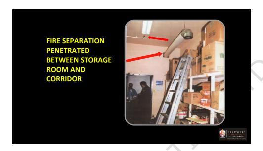
For heating purposes the fire separation between the corridor and the storage room has been penetrated. A fire starting in the storage room will quickly spread to the exit corridor on the other side of the wall. In this case a sprinkler head is located in the storage room which will help contain the fire in the room but the fire separation has been breached and proper fire separation with fire stopping materials should be installed to prevent the spread of fire.
