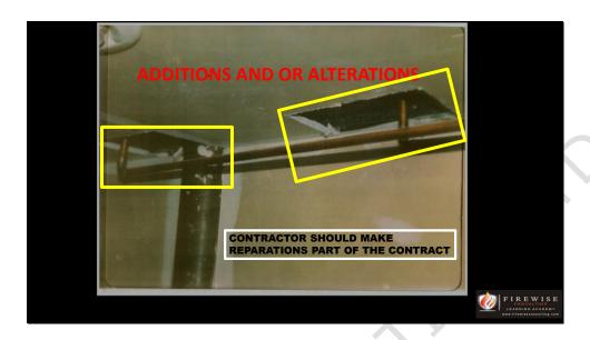
In this case water lines are re-routed by a contractor but the holes in the fire separation were never repaired. A fire in this room would quickly spread into the concealed space creating a significant suppression problem for firefighters. The people performing the renovations should be required to repair fire separations as part of the contract.
