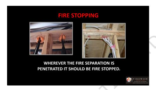
Wherever the fire separation is penetrated it should be fire stopped. When having repairs or alterations done to the building the owner should specify that fire stopping is required as part of the job. Qualified trades people know that fire stopping must be provided in fire separations and around pipes and wires that penetrate a fire separation but often they exclude that from the contract. The building owner or manager should insist fire stopping be completed properly.
