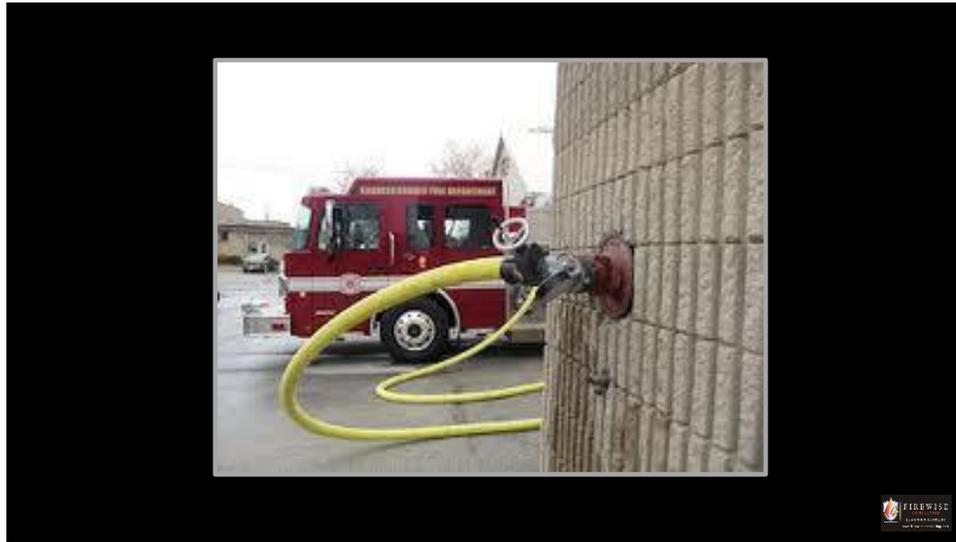
The fire department connection should be located on the street side of the building and be fully visible and kept unobstructed at all times to ensure immediate access. It should be located so the fire engine and its hose lines do not obstruct access to the building for other apparatus when connected to the FDC.
