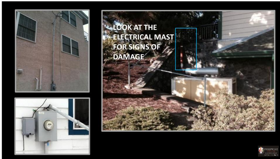
Look at the electrical mast for signs of damage. In the picture on the left why is the wire hanging down? It is better to identify and fix the problem now rather than waiting for an emergency.
