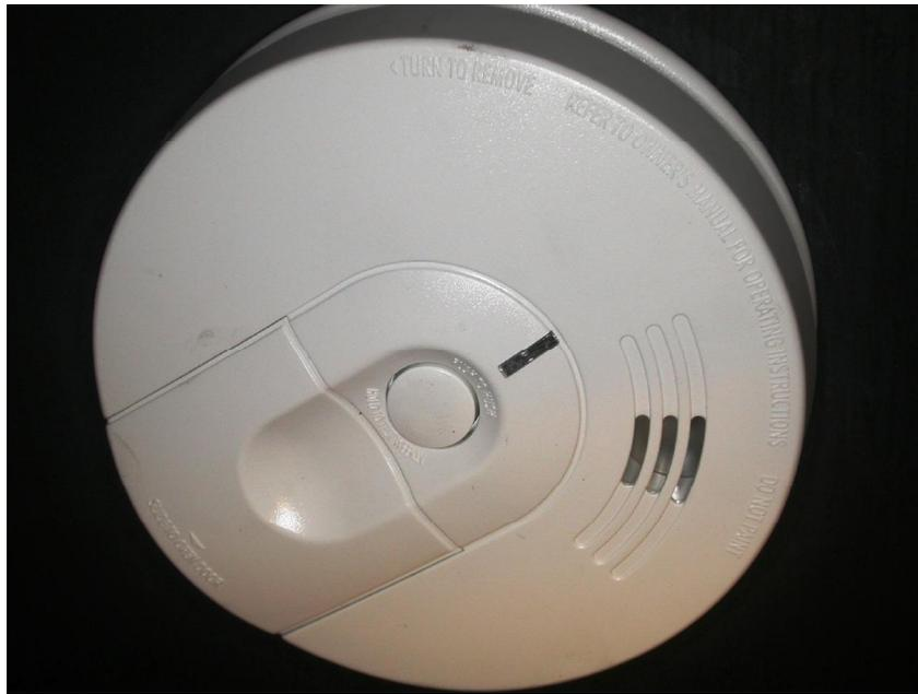
**Figure 20.3** This figure shows the cover of an FACI alarm that sounded during exposure to a smoldering cable fire.
