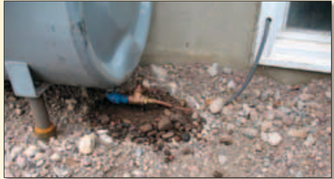
Small spill from a leaking valve.
