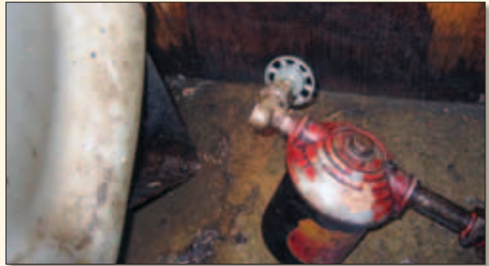
Broken valve on oil tank in basement.
