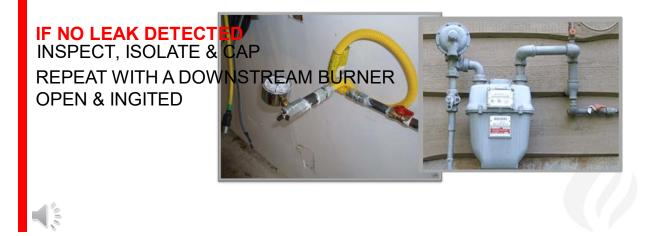
Fuel gas systems are designed to retain moderately pressurized gas. The presence of leaks in the system can be determined by detecting a drop in pressure within the closed system. Before the piping is used for testing, the system must be inspected and any obviously damaged portions of the system should be isolated and capped. Sometimes it may be necessary to test the piping in multiple sections due to physical damage to the system.
