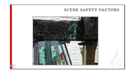
In this case, the fire investigator needed to remove a heavy beam due to the potential for collapse. Before removing the beam with heavy equipment the fire investigator marked the beam with spray paint showing which way was up and which side faced the fire so that it could be replaced later in the investigation if it became necessary. This would also assist other investigators that may attend the scene later.
