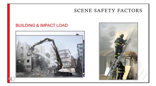
An impact load is a sudden added load to a structure. For example, when a fire fighter jumps off a ladder onto a floor or roof, or when part of the building collapses on to another part of the building. If the structure is already weakened this can cause it to collapse.
