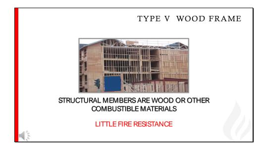
Type V – Wood Frame construction buildings have structural members made from wood or other combustible materials.
