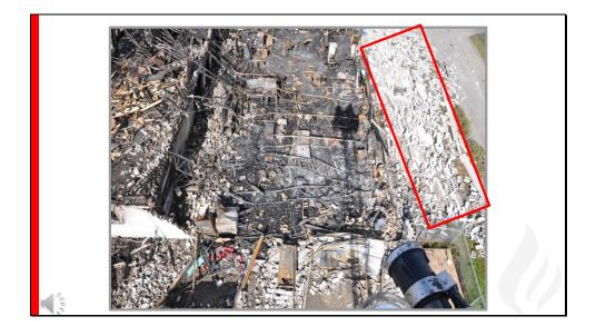
This aerial view of the building after the fire reveals remnants of the metal roof trusses and the masonry wall that collapsed is outlined in red.
