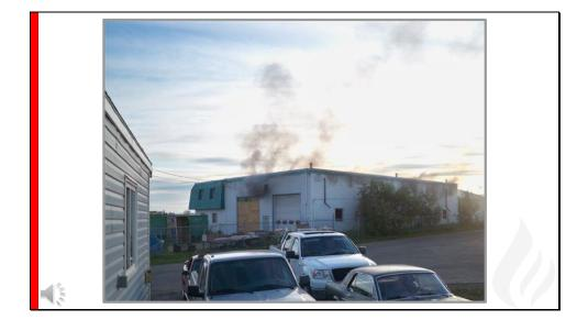
This small warehouse is an example of how quickly exterior walls can collapse when the metal roof structural members are subjected to intense heat.
