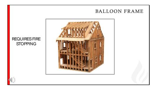
In balloon frame construction, the studs go from the foundation wall to the roofline. This type of construction is typical in many homes built prior to 1940. They were built without fire stopping, allowing a fire that has developed in the wall to rapidly extend into the attic.
