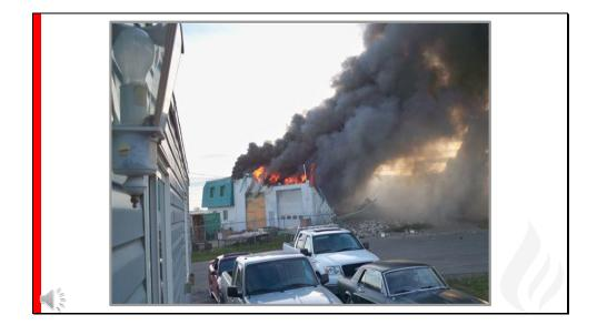
As the fire inside the building developed metal trusses expanded with enough force to cause a masonry wall to collapse.
