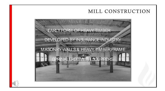
"Mill" construction was an early form of Timber Frame construction developed by the insurance industry. They often had masonry walls and heavy timber frame. Generally they were sprinklered with scuppers in the side walls of the structure, for purposes of draining water. The scuppers are usually placed at or near floor or ground level, and allow water to flow off the side of the open-air structure, instead of pooling within the walls.
