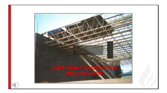
Lightweight roof trusses are generally used in lightweight commercial construction. These types of roof systems are flat with plywood on top of the trusses to give added strength with a weatherproof membrane over the plywood.
