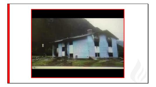
Note the fire starts in the basement room on the Alpha Delta corner. The pressure front takes the siding off the house in large pieces which is typical of low order damage. The flame front moves through the basement and main floor but goes out.
