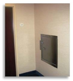
Refuse and linen chutes must be constructed to prevent the spread of fire products, including fire-resistive opening protectives, as illustrated here from an older version of a building code. Openings into corridors are not permitted in current codes.
