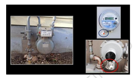
Identify the location of the utility connections such as gas and electric meters. Most jurisdictions require tamper seals on both gas and electric meters to ensure that they have not been tampered with. They are made of nylon monofilament line at least 0.644 mm or a metal 14 gage wire. Check to make sure that tamper seals are in place and not broken.
