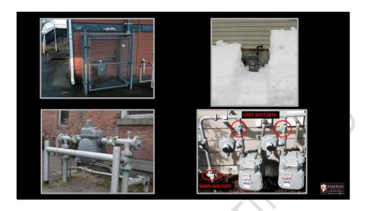
There must be adequate collision protection for utility connections. Metering and regulating equipment must be protected from potential physical damage. Where there is potential for vehicular damage including forklifts and other moveable equipment, a vehicle barrier or fencing should be provided.
