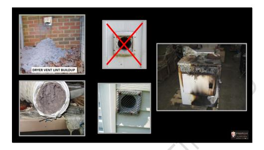
Look at the vent outlets on the exterior of the building to make sure they are in good repair. They should be equipped with a cover to prevent foreign material from entering and blocking the vent. Check to see if there is any buildup of combustible products such as lint from clothes dryers. If lint is visible at the outlets it can be assumed that the vent needs cleaning. A clogged vent can result in a dryer fire or dryer and vent fire which could be devastating.
