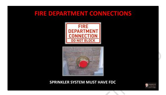
Buildings equipped with an automatic sprinkler system must have a fire department connection on the outside of the building easily accessible by the fire department.
