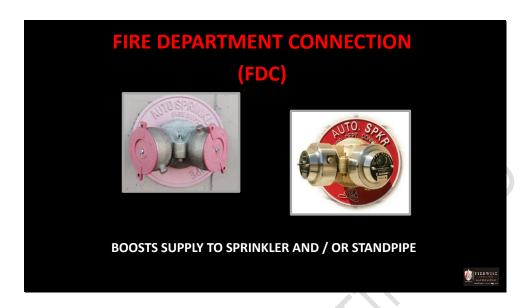
If the building has an automatic sprinkler system or a standpipe and hose system there should be a Fire Department Connection or FDC, on the outside of the building. When a fire occurs, water is discharged from the sprinkler heads to suppress and extinguish the fire. The fire department connection is used by the fire department to supplement the water supply to the sprinkler or standpipe and hose system.
